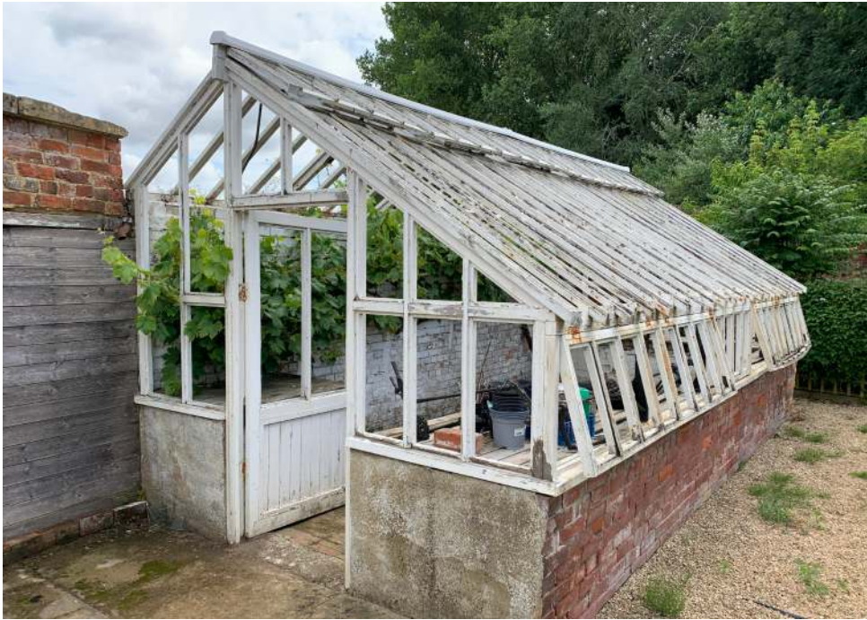
Figure 7D Existing greenhouse gable end condition.
