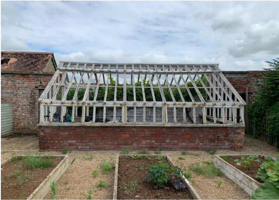
Figure 7C Existing greenhouse condition.
