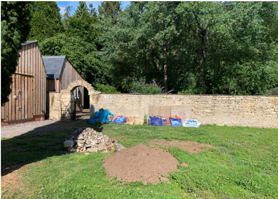
Figure 7B View to the west of the existing wall against which the potting shed and covered store will be constructed and the greenhouse relocated.
